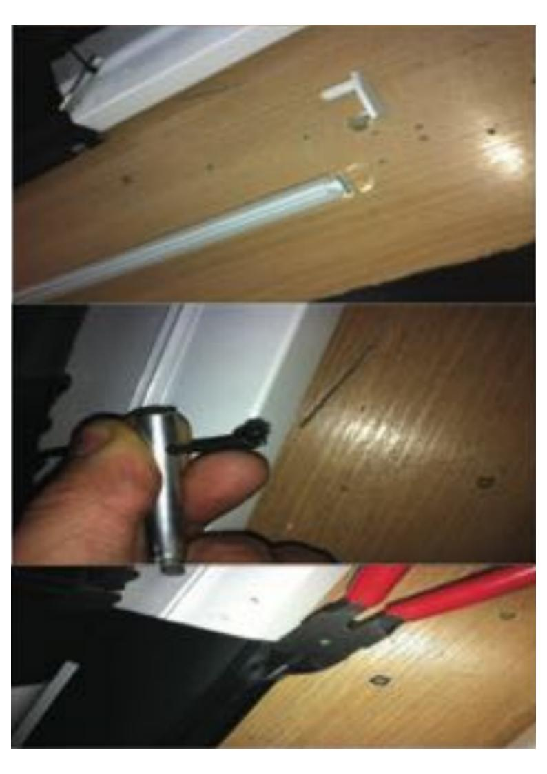
f) Replace the plastic adapter which is on the left side in old roll and put it to the new roll, than install the new roll.
