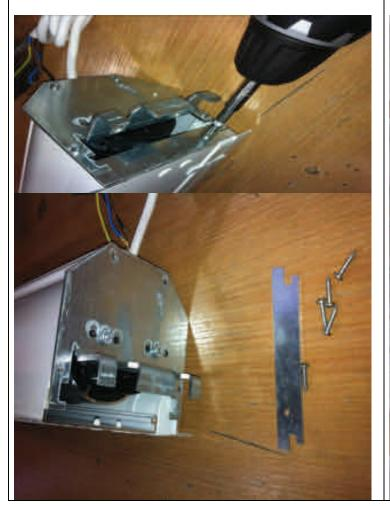
d) Open the top part of the casing. Pull back into the casing motor cable and then remove the motor from the roll.
