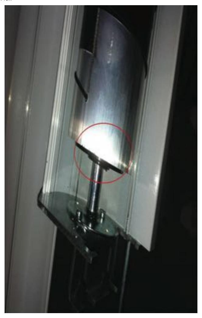
g) Inside the welding of fabric put the iron bar and secure it with metal clips, then slide carefully the batten into the fabric welding. Install two metal pins and make new nodes on the rubber strings.
